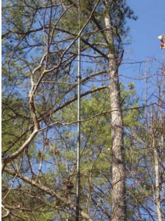
Completed antenna project. 45' tall guyed 1.75" aluminum tubing mast.
